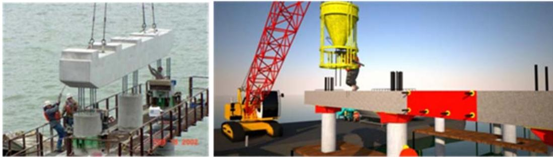
Figure 7 Erection of Precast Pile Cap, (a) Erection Precast Pile Cap, (b) Pile Cap Closure
