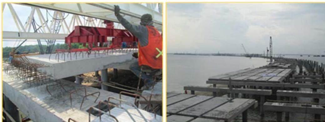
Figure 8 Erection of Precast Slab, (a) Erection Precast Pile Cap, (b) Joint Slab Casting
