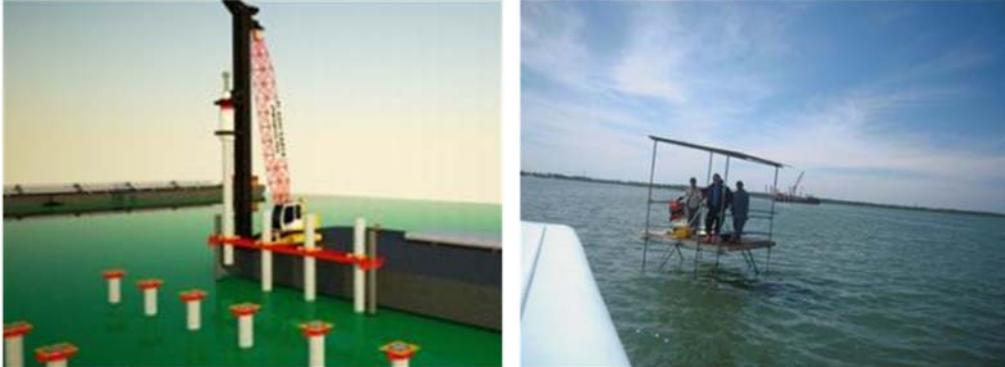
Figure 4 Installation of Prestress Concrete Pile , (a) Pile Installation in the Middle of the Sea, (b) A Semi Permanent Bench Mark in the Middle of the Sea
