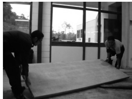
Figure 3: Two workers lifting a 2.4 m PSSDB floor panel
