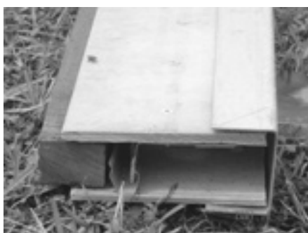
Figure 4: Double skinned wall panel with window openings
