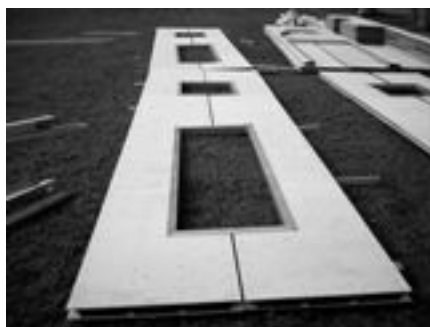
Figure 4: Double skinned wall panel with window openings
