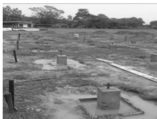
Figure 8(a). Construction of footing
