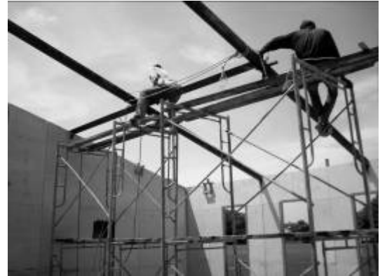
Figure 9(a): Erection of rafter
