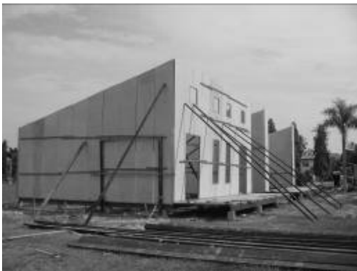
Figure 8(d): The propped wall and laid floor panels
