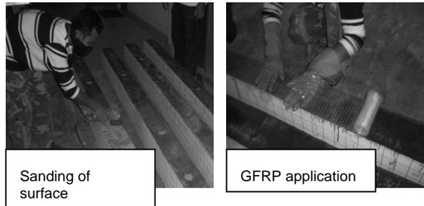
Figure 3 Application of GFRP Sheet
